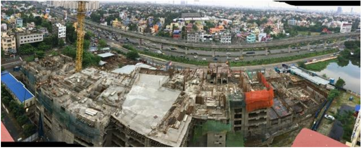
Avidipta Ph - 2 Project as on Progress
